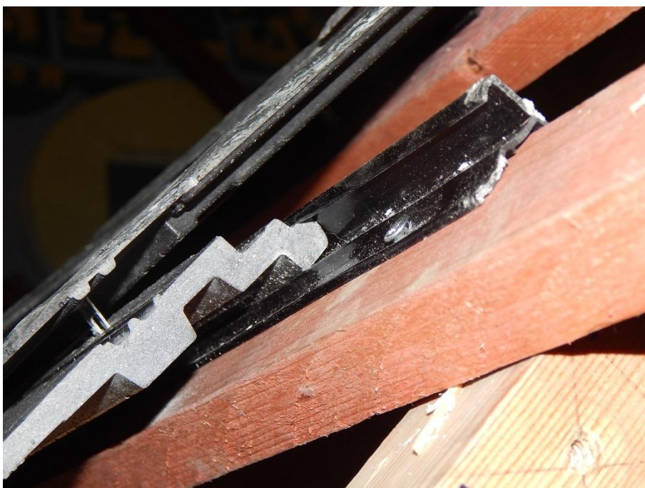
Figure 5 Integral clip disengaged from slate below
